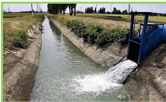
Picture 4. Melioration channels reinforced slopes.
